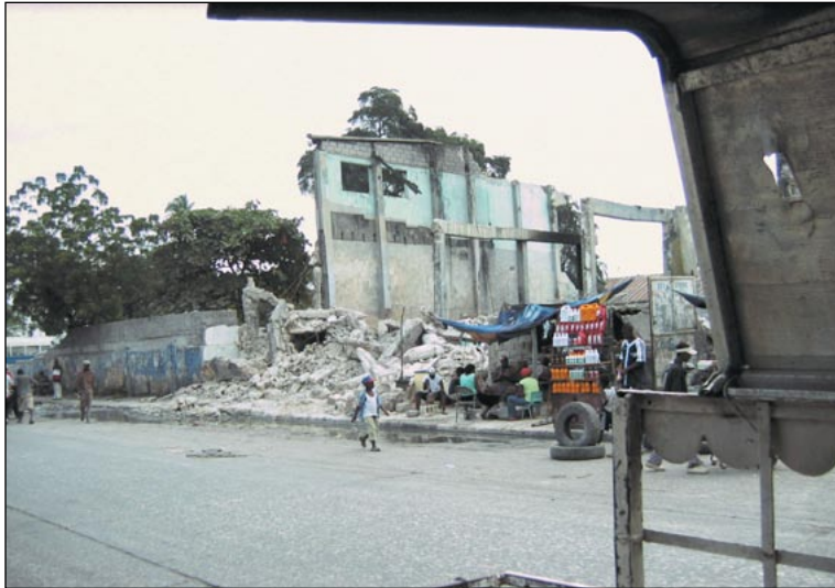
A Young Boy Walks Alone on the Road after the Earthquake in Port-au-Prince.
